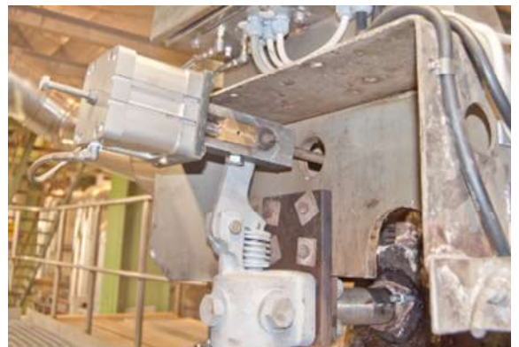
Local actuator on sootblower poppet valve
